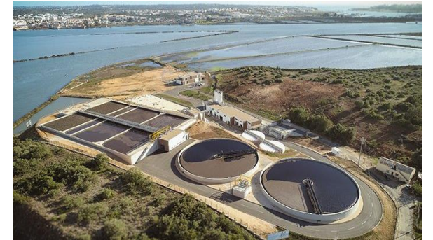
Waste water treatment plant
